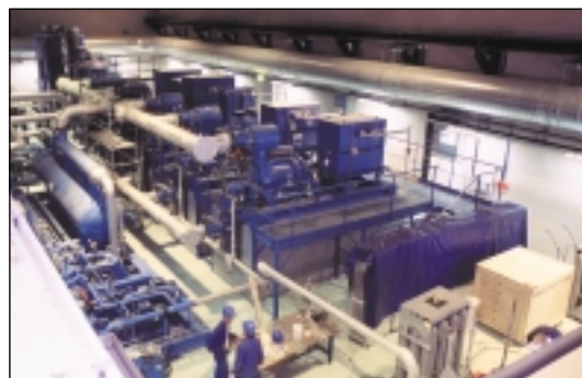
Helium compressors at the test and assembly area for LHC equipment.
